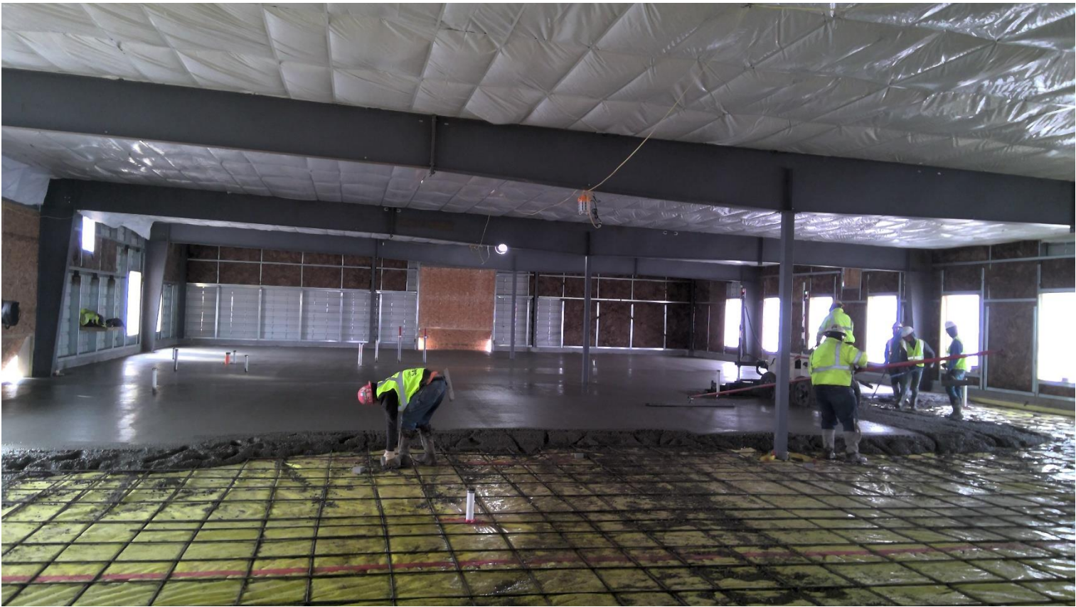
Pouring the concrete slab in the classroom wing.
