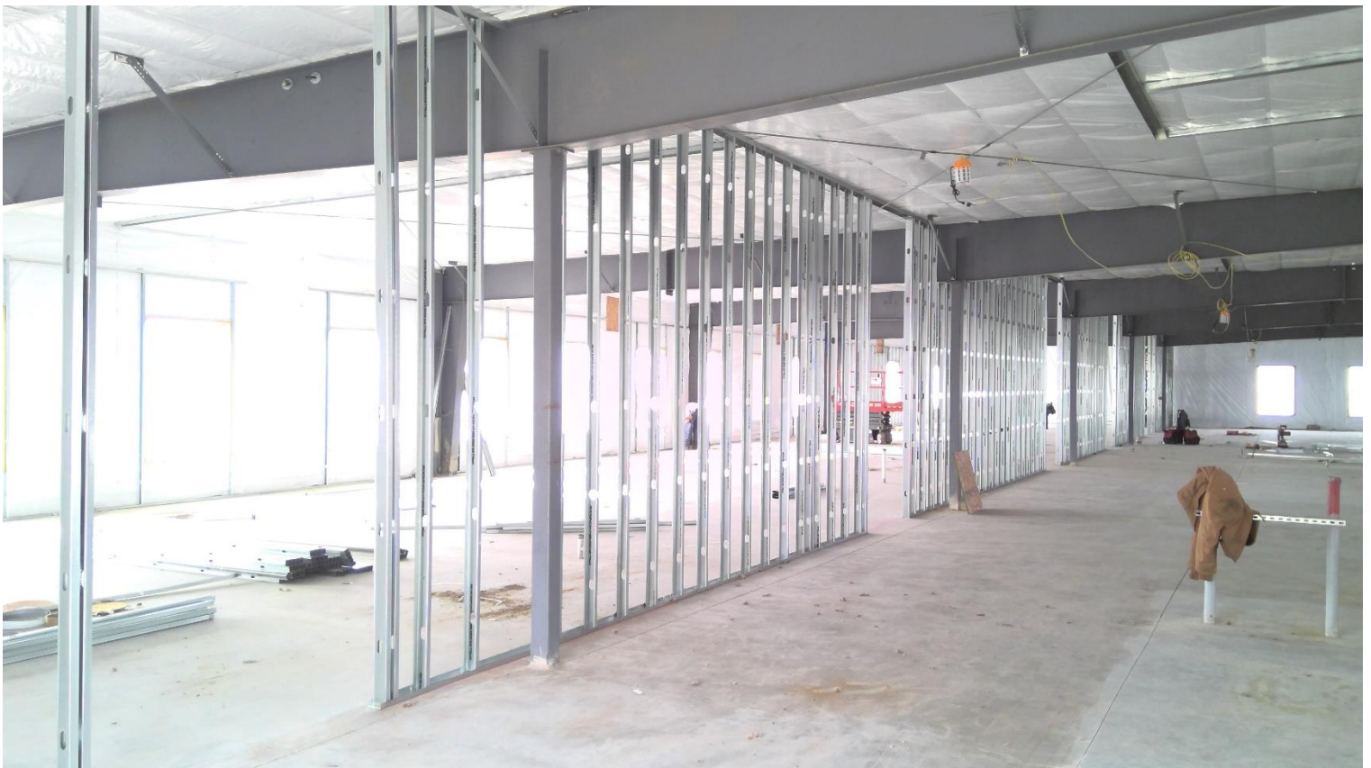
Steel stud walls in the classroom corridor.
