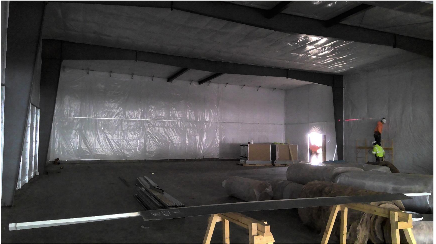
Steel stud walls in the gymnasium.
