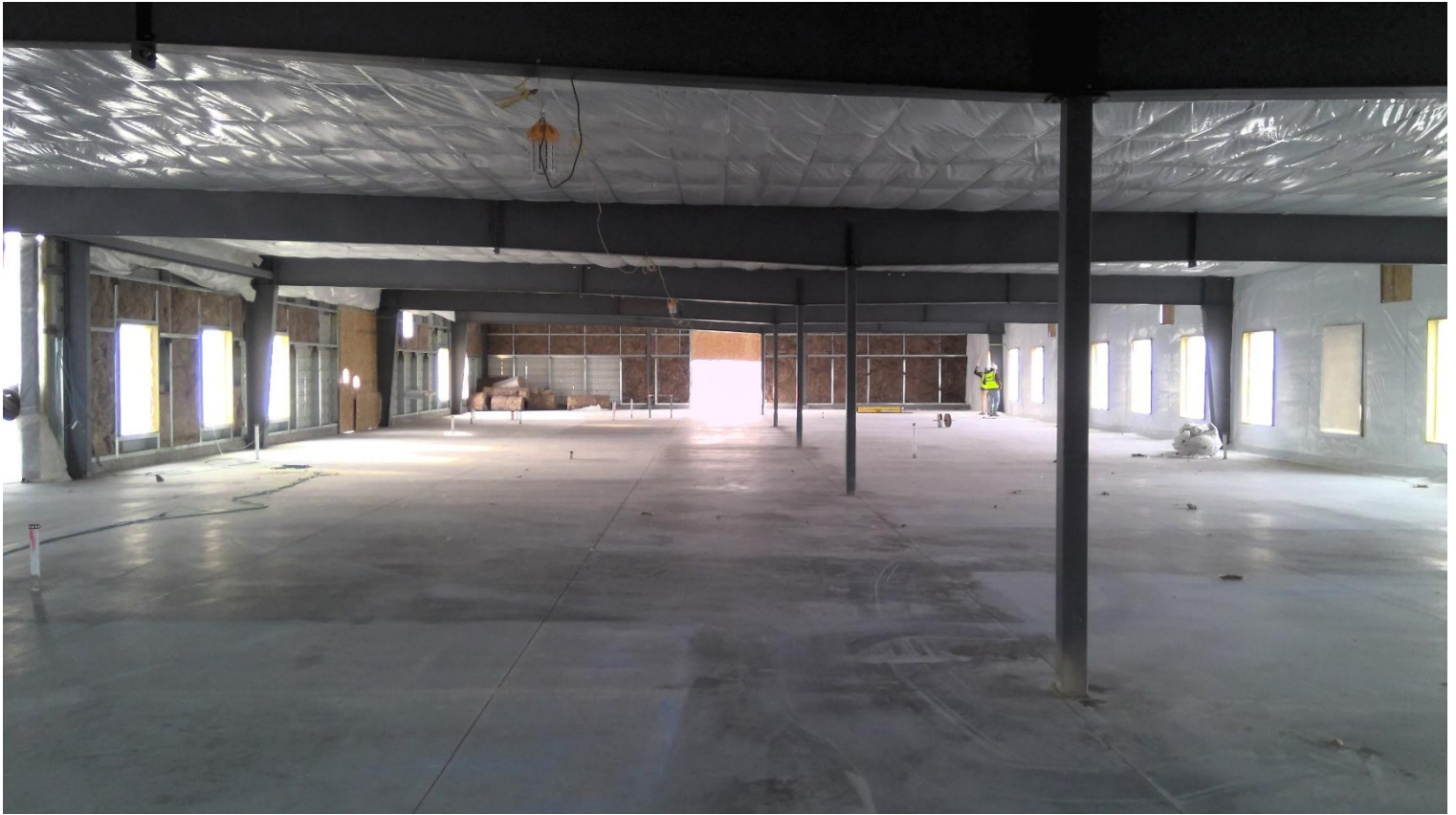
Sealed concrete in the classroom wing.
