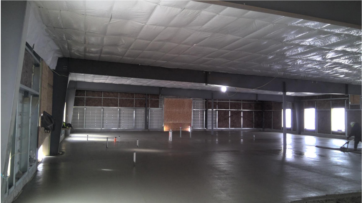
Screeding off the concrete slab.
