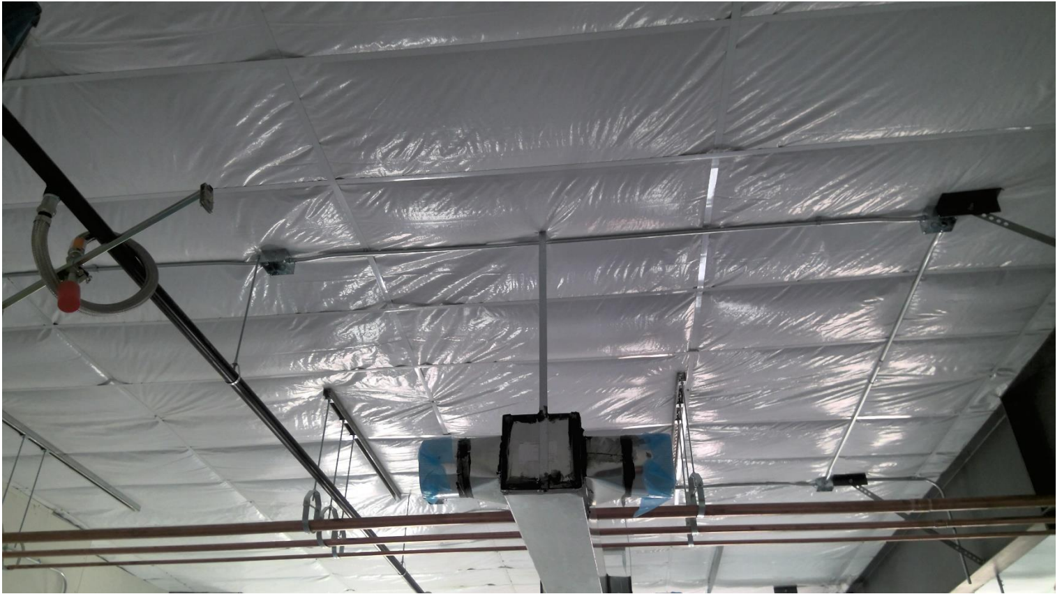
Installing overhead electrical conduit and water piping.
