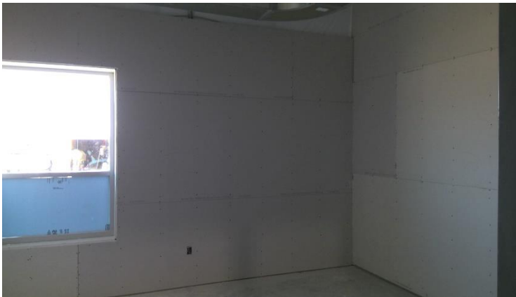
Sheetrock inside of classrooms complete.
