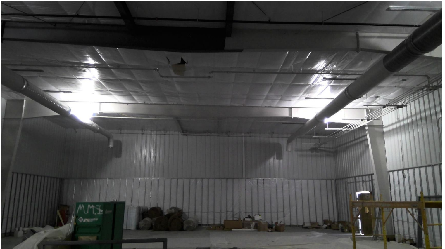
Painting ductwork and structural steel in the gym.
