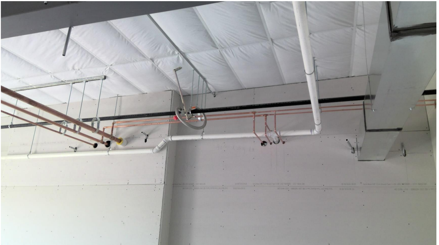
Installing overhead water piping and vent piping.
