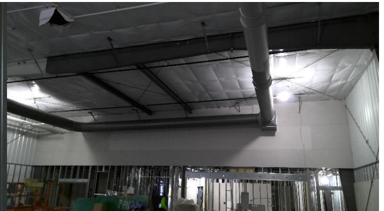
Sheetrock for mezzanine complete.
