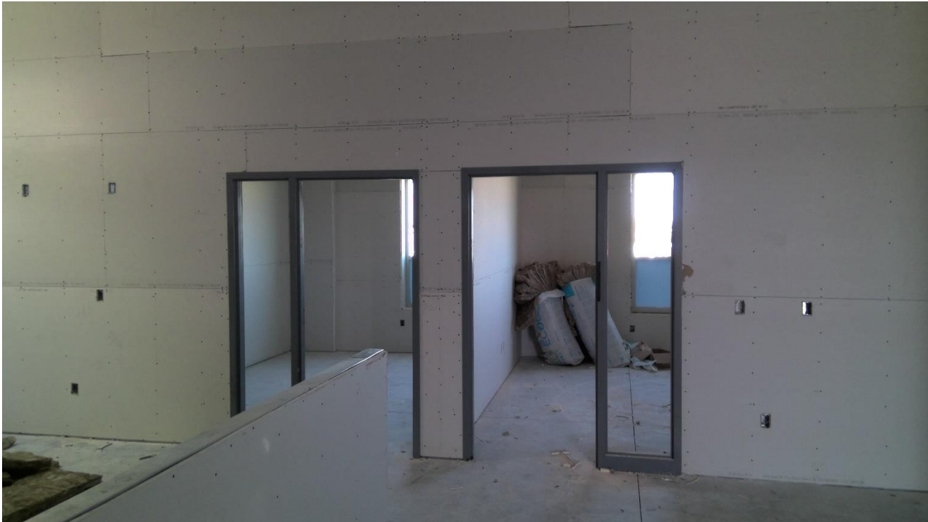
Sheetrock in office areas complete.
