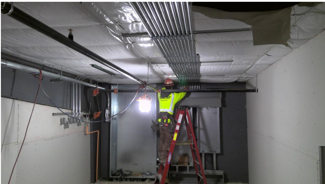
Installing conduit to the main electrical panel in the mezzanine.
