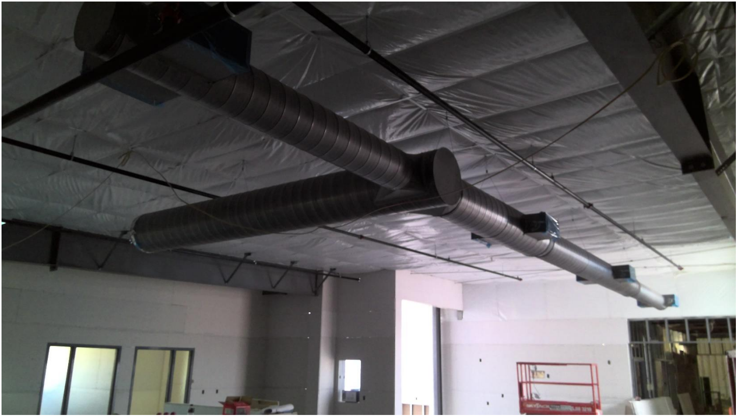
Installing duct work/ painting or insulating duct work.
